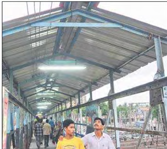
The pedestrian bridge at Vidyavihar station is getting a metal roof. The platforms (below) continue to have asbestos roofs
